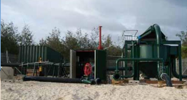
*Pipeline booster station operating at Noosa, Queensland (SlurrySystems)*
